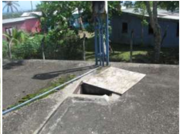
Reservoir inlet lids are missing
