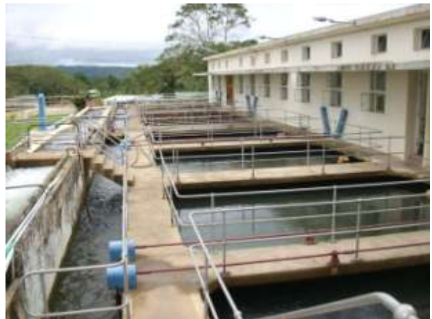
Rapid sand filters-Tamavua Plant
