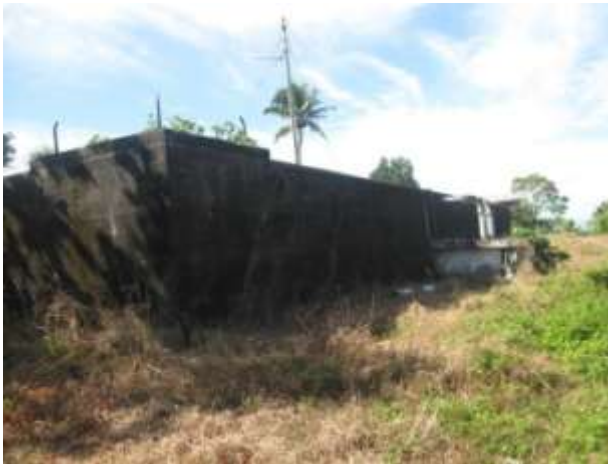
Concrete Reservoir- Nagatugatu -unmaintained
