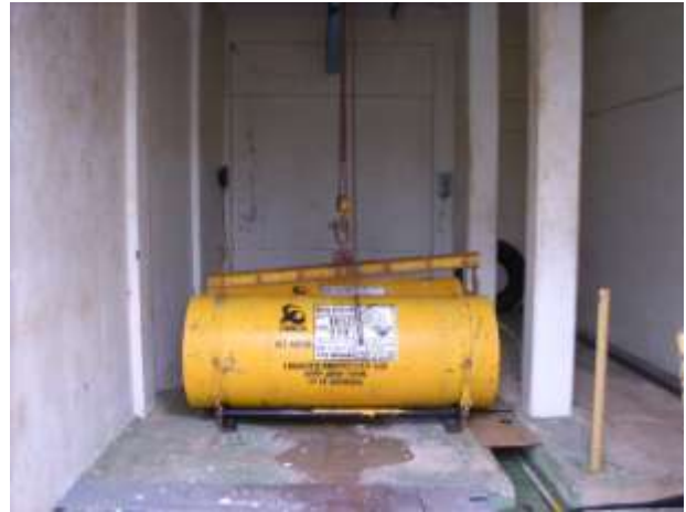
Gas chlorine cylinders -920 kg
