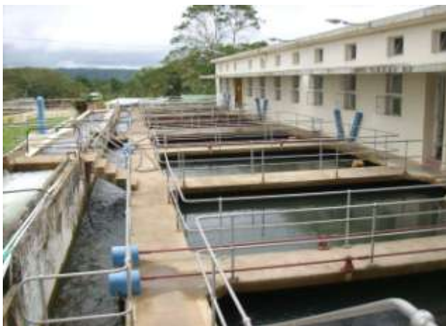
Rapid Sand Filters 8 –Tamavua Plant
