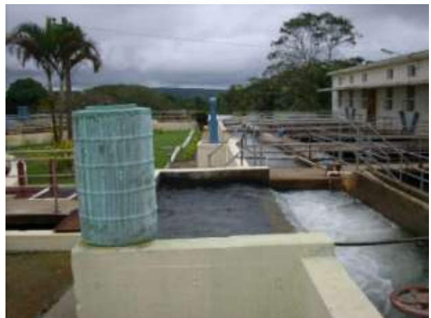
Addition of Copper sulphate /Alum/Soda
